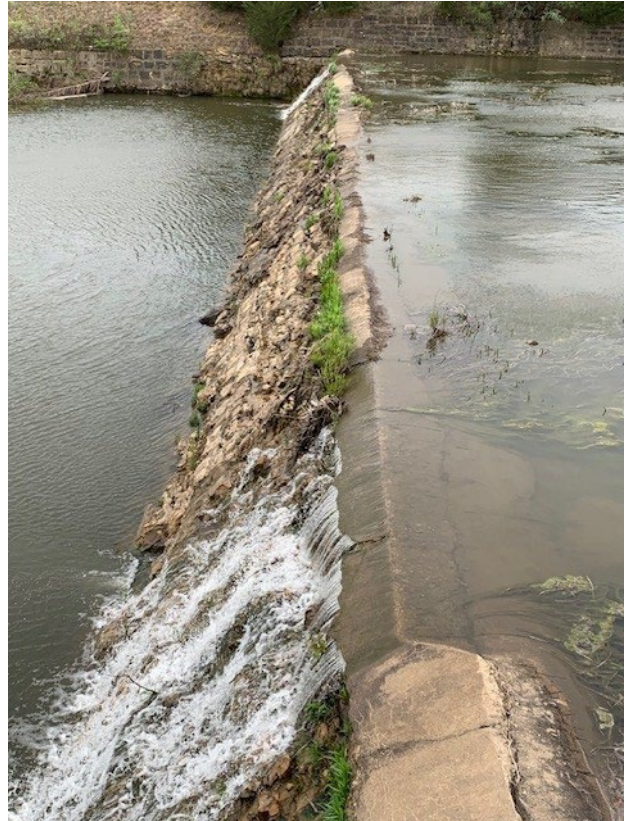
Pic. 2 – Spillway drop-off.
