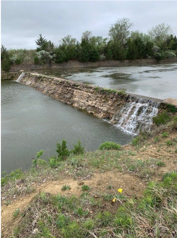
Pic. 1 – Spillway drop-off.
